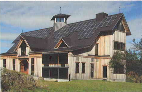
Teal Farm's 12,000-square-foot Energy Barn is designed to gather and distribute energy from five different sources: wind, solar, solar thermal, microhydro, and biomass.
